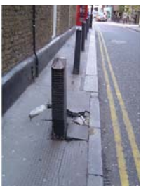
Damaged City Bollard and footway on Shelton Street.
