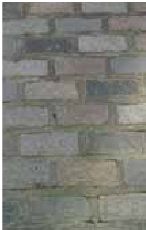
Detail of dressed multi-coloured flame setts - Monmouth Street.
