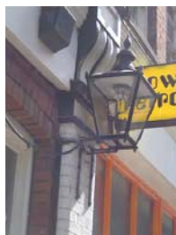
Detail of wall-mounted Windsor Lantern.
