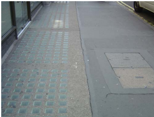
Long Acre - The relationship between cellar lights and the footway is often crude. A more sensitive approach (e.g. a trim of York stone setts) would make a more attractive solution.
