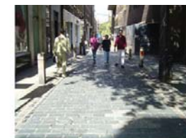
Reclaimed Granite sett carriageway - Neal Street.
