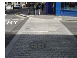
Dressed Granite sett vehicle cross-over - Endell Street.
