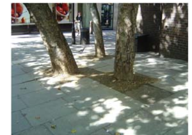
Footway at Neal Street junction is being dislodged through tree root growth.
