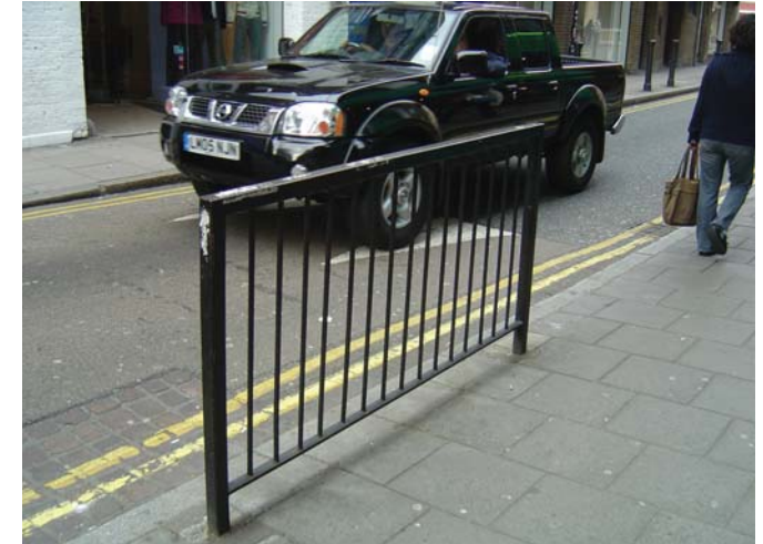
Shelton Street - Guardrail can cause an unnecessary physical obstruction and add to visual clutter. This is particularly noticeable on Shelton Street.
