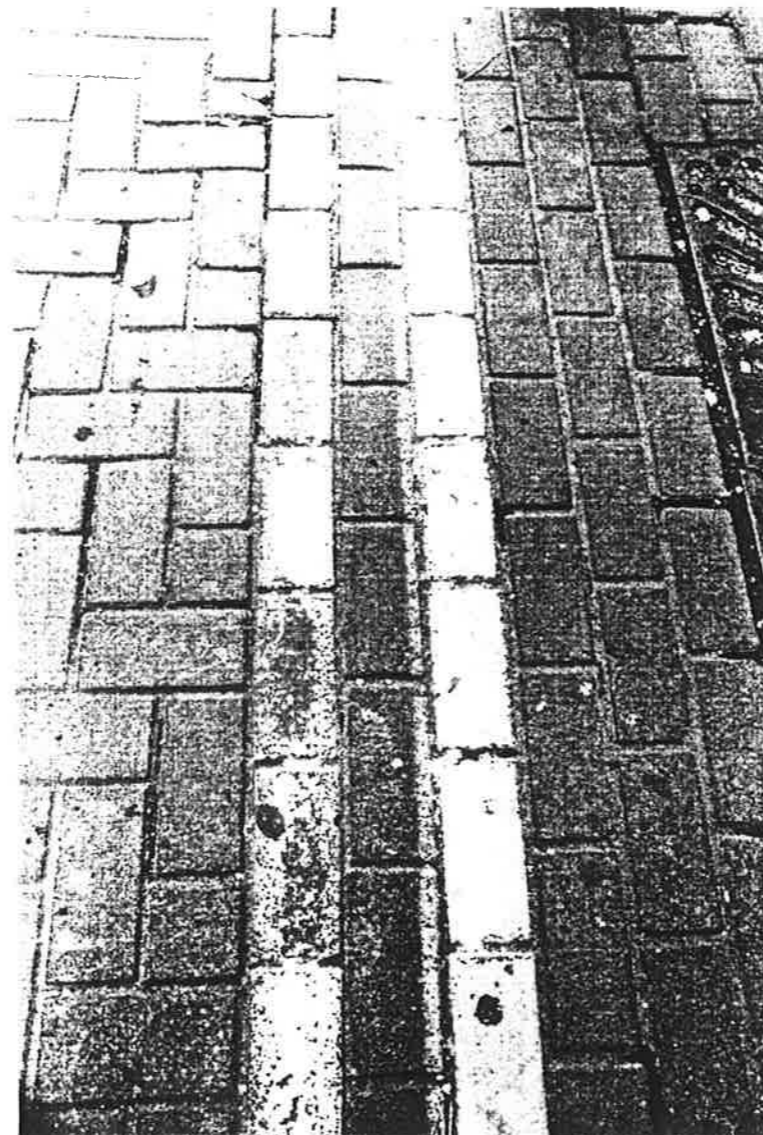
CONCRETE BLOCKS IN MODERN HERRINGBONE PATTERN
