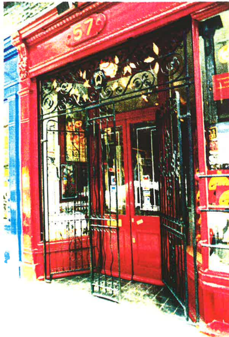
RESTORED SHOP FRONT IN MONMOUTH STREET
