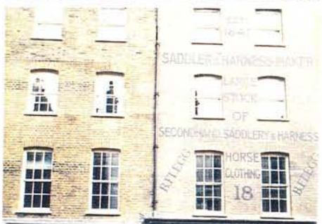
Examples of some of the many types of brickwork in Seven Dials.
