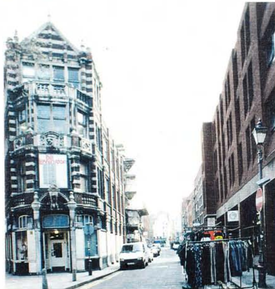
Properties in Earlam Street were threatened with redevelopment. The guidance in the draft version of this document helped ensure a scheme of sympathetic improvement.
