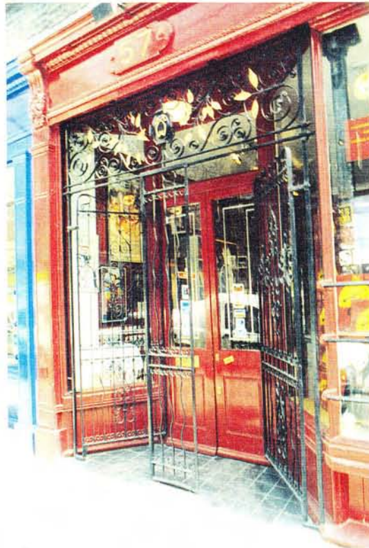
Restored shopfront in Monmouth Street.
