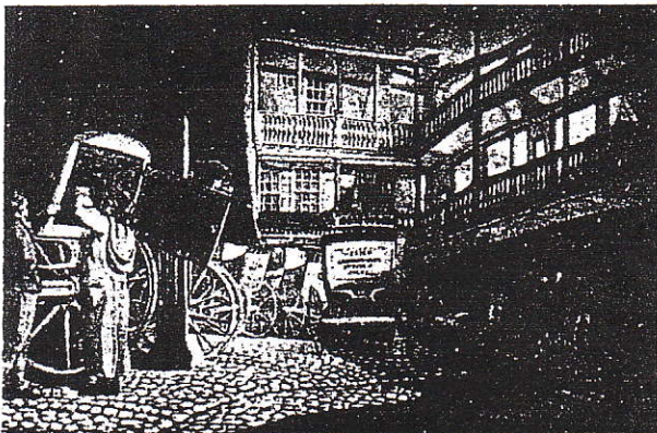
Figure 3 Schnebbelie The Yard of the Spread Eagle, Gracechurch Street (1814). Small pebbles with drainage channels. Leadenhall Market is now on the site.
