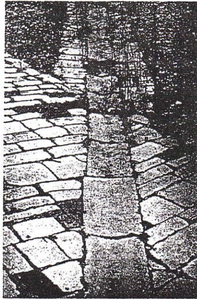
Figure 11 Hare Court, Inner Temple, detail of Purbeck drainage channel, 11 inches wide with 1-inch dishing.
