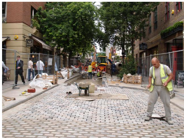
Monmouth South Works – the colour of the grout can significantly impact on the overall appearance
