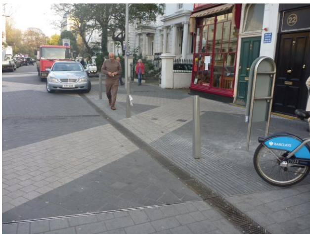
Exhibition Road – granite setts across the carriageway and footway achieve a unified aesthetic
