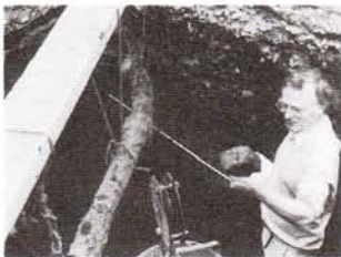
Architect, 'Red' Mason, inspecting the extensive 1693 foundations, which were revealed when digging the first trial hole.
