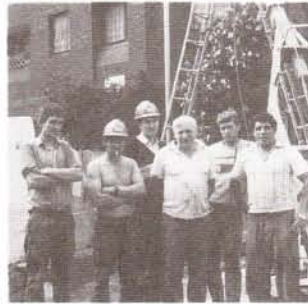
The Foundation Site Team are pictured in front of the Piling Rig with the Tunnelling Team on the left and the Piling Team on the right.
