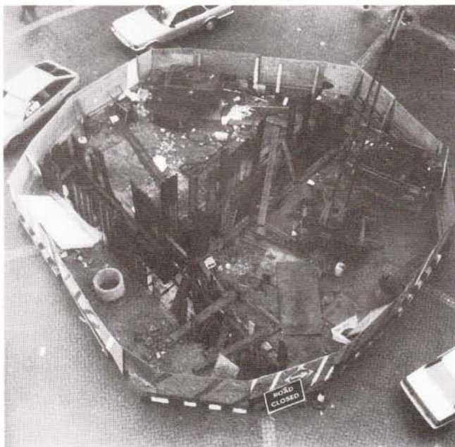
Aerial photograph of the final stage of the foundation works showing the T-shaped holes for the beams in the same form as the diagrammatic plan.
