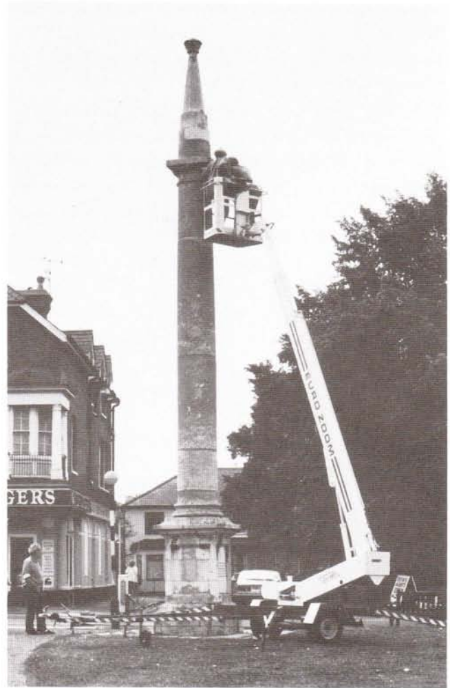
The Architect inspecting the Capitol of the Weybridge Column.
