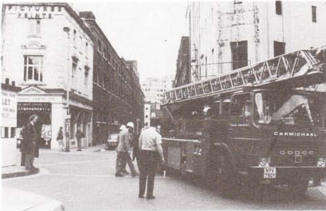
Borrowing a Fire Engine. To ensure that the foundation works could be carried out with minimal traffic disruption the Soho Firestation lent us their largest vehicle for an afternoon. It is pictured with representatives from the London Borough of Camden Planning and Works Department, the Metropolitan City Police, Whitfield Partners, Taylor Woodrow Construction Ltd etc.
