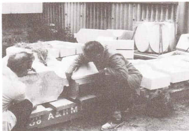
Architect 'Red' Mason and Works Supervisor Alan Watts, at Ashby & Horner Stonemasonry, checking the cornice to the pedestal against the zinc template.
