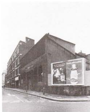
The old Central Electricity Generating Board Station at West Street in 1973. Demolished by the Greater London Council to provide housing in Earlam/West Street.
