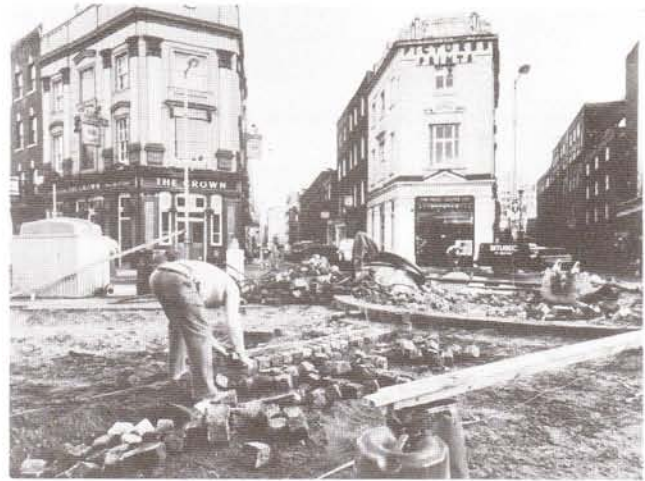
Reparing Seven Dials. Camden Council, with D.O.E. support, completely re-surfaced the Dials with pavoirs, cobbles and bollards, and created a central island in preparation for the reconstruction of the Sundial Pillar. This was part of an extensive programme of environmental improvements around Seven Dials which has involved tree-planting, pavement widening and traffic management.
